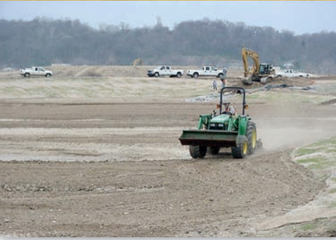
Site preparation for wetland mitigation, Cincinnati, OH
