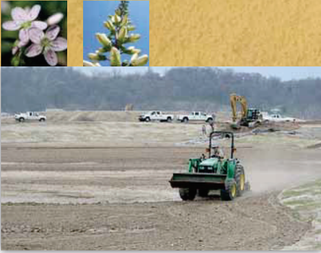
Site preparation for wetland mitigation, Cincinnati, OH
